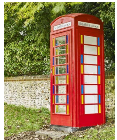
K6 Kiosk at St James church Woodmancott
