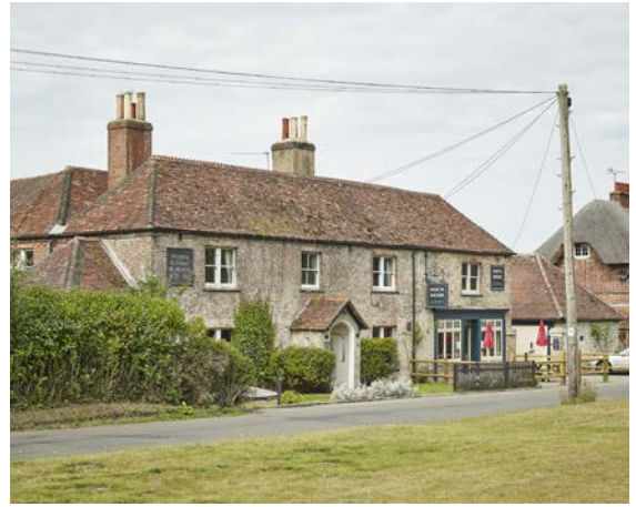
Northbrook Arms, East Stratton
