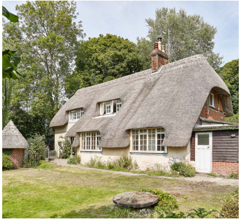
Old Mill Cottage
